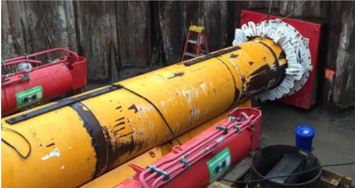
Figure 2: Direct Pipe® Set-Up at Ground Entry.
