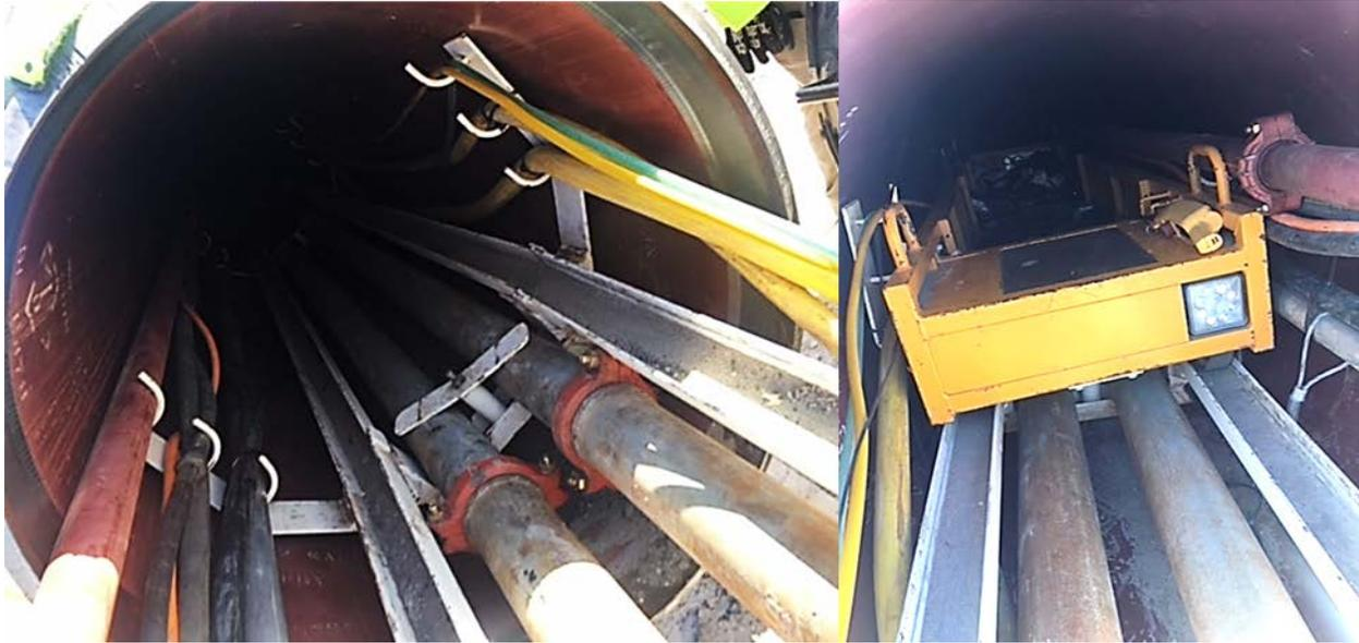
Figure 4: Interior Pipe Rail and Umbilical Configuration.
