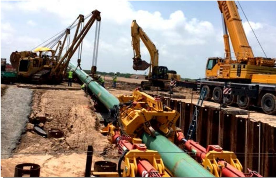
Figure 6: Direct Pipe® Tunneling Operations
